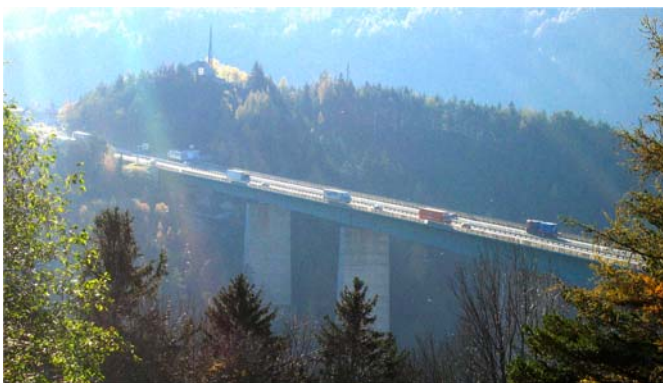
Fig. 3 An endless caravan of heavy trucks crosses the Austrian “Europabrücke” on a late autumn afternoon. The viaduct is part of the Brenner traverse between southern Germany and northern Italy.
